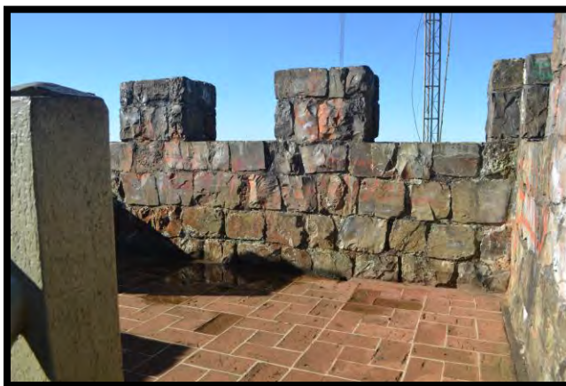
Photo 8. Observation area at the top of the tower.
