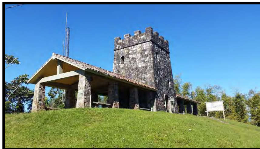
Photo 5. View of the Observation Tower facing southwest.
