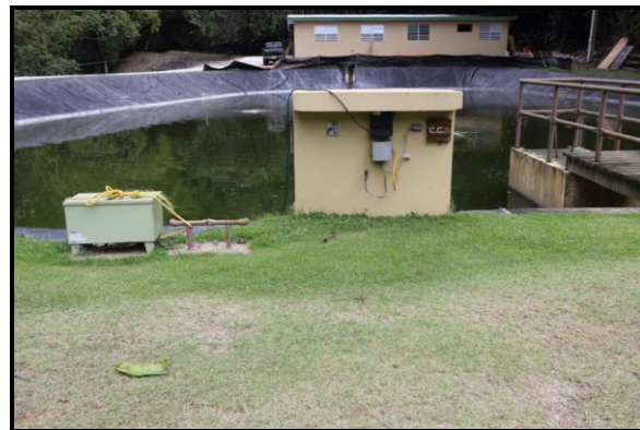
Picture 41 and 42. View of the grow-out pond #6 looking southeast (#41) and looking northwest (#42). In the first picture has a close up view of the impermeable membrane used to cover the bottom and sides of the pond. In the background of second picture is the Equipment Storage Building.
