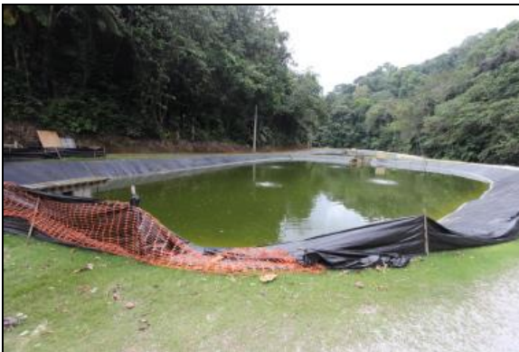
Picture 41 and 42. View of the grow-out pond #6 looking southeast (#41) and looking northwest (#42). In the first picture has a close up view of the impermeable membrane used to cover the bottom and sides of the pond. In the background of second picture is the Equipment Storage Building.
