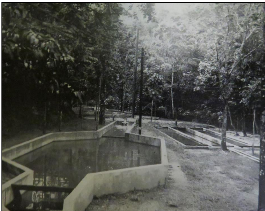
Figure 10. View of the holding tank and in the background the retention tank and circular tank. Revista de Agricultura y Comercio de Puerto Rico. Marzo 1939
