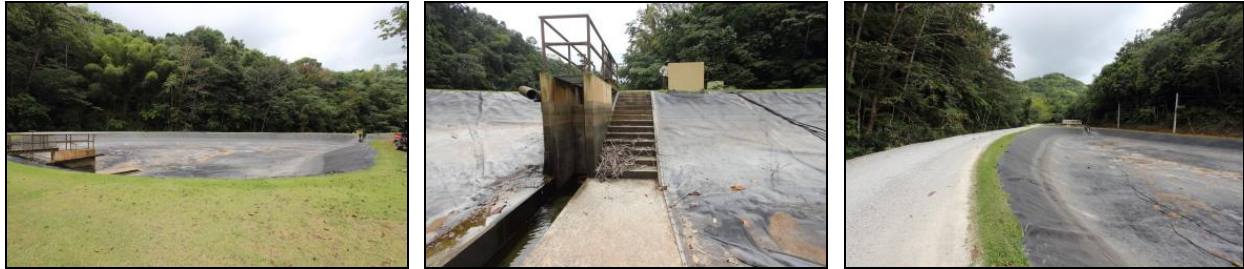
Picture 27, 28 and 29. Views of the grow-out pond #4 (CC4) emptied for routine maintenance. The photos were taken from the interior service road, close up of its fish kettle and from the exterior service road (close to the river bed).
